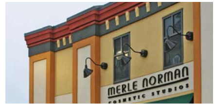
Figure 18.17 Goose-neck lights mounted above signage reference allow the branding elements to stand out from a distance.
