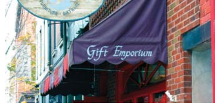
Figure 18.13 An example of a semi-permanent fabric awning that incorporates signage.
