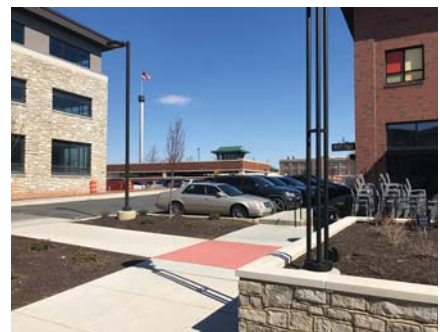
Figure 20.5 Parking lots located behind corresponding buildings allow ease of access to businesses but emphasize pedestrian-scaled storefronts.
