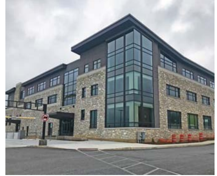
Figure 15.42 Examples of commercial buildings that use vertical articulation to visually break down the scale of the building.
