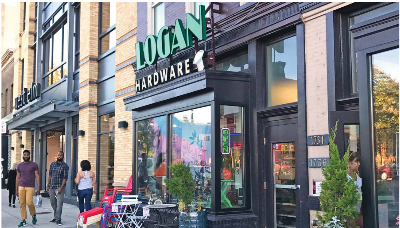
Figure 18.12 An example of an open, transparent, and low-reflective storefront opening that is vibrant and inviting.
