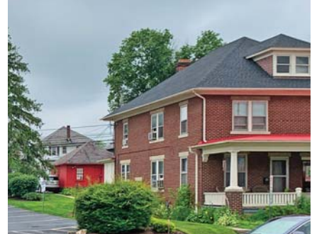
Figure 20.8 Referencing similar architectural elements creates visual continuity between primary and accessory structures, which are typically accessed from alleys and conceal unattractive uses from pedestrian routes.
