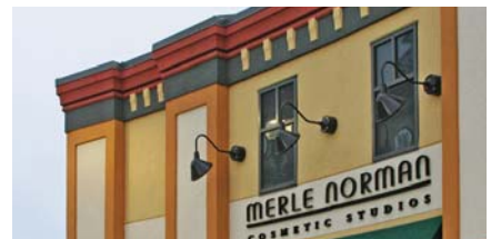
Figure 18.17 Goose-neck lights mounted above signage reference allow the branding elements to stand out from a distance.
