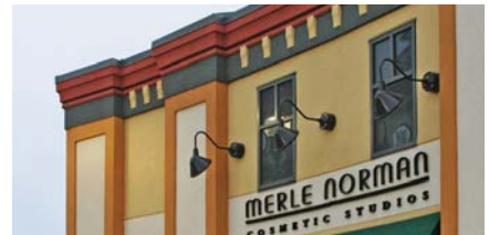
Figure 18.17 Goose-neck lights mounted above signage reference allow the branding elements to stand out from a distance.
