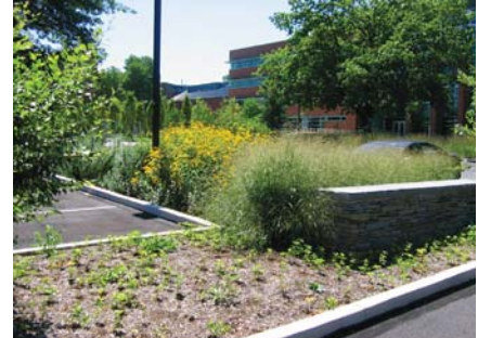
Figure 20.6 An example of lush plantings in parking islands that collect and absorb stormwater in an institutional context.
