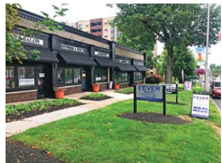
Figure 20.2 Walkways connect private and public realms.
